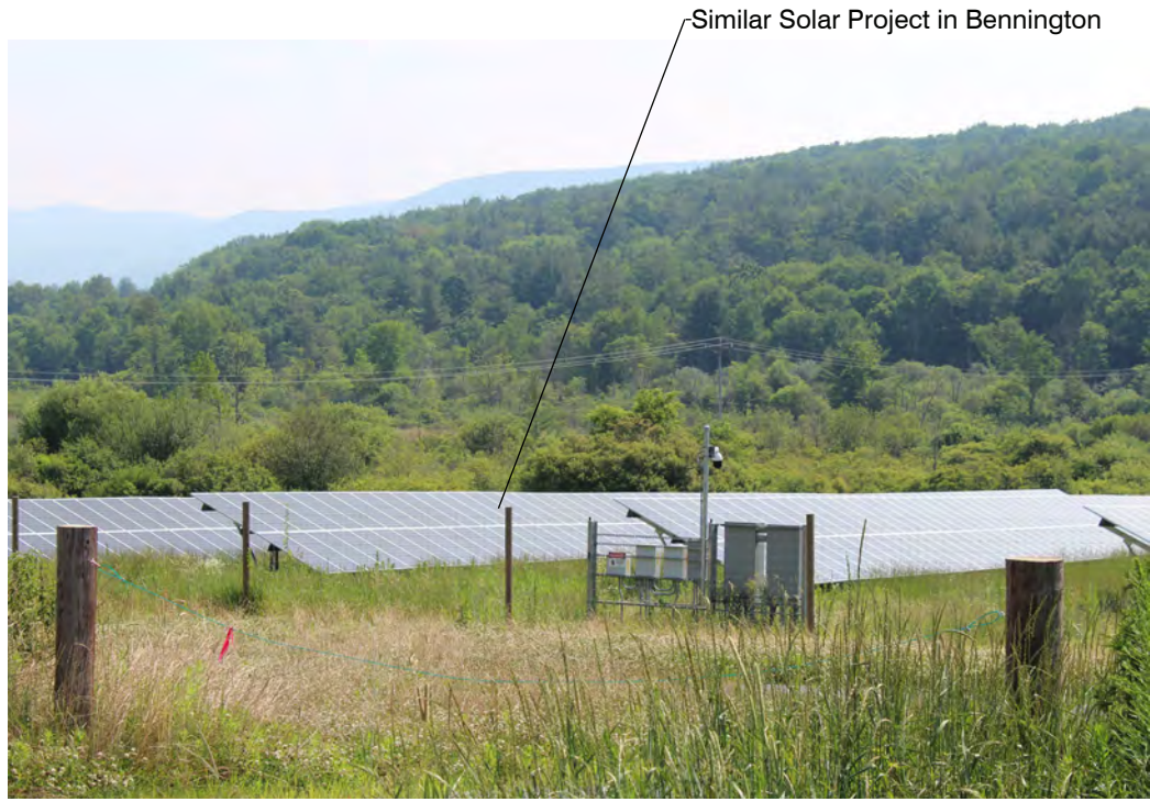
E - VIEW LOOKING NORTHWEST FROM ROUTE 7 TOWARD SIMILAR SOLAR PROJECT
