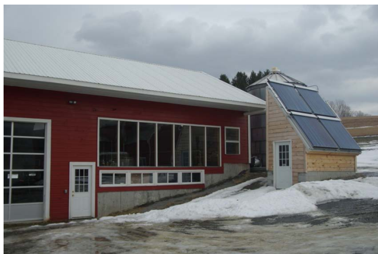
State Line Farm in Shaftsbury produces biofuels at this modern facility; the evacuated tube solar collectors on the right of the picture provide heat for the building and grain processing.
