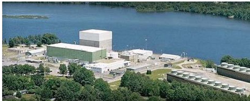
Vermont Yankee produces 650 MW of electricity, meeting about one-third of the state's demand.
