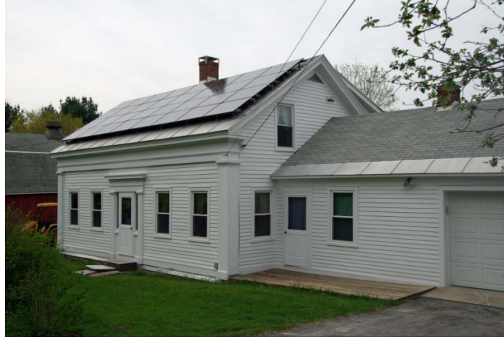
The photovoltaic array on the south-facing roof of this house in Bennington provides most of the electricity used in the home.
