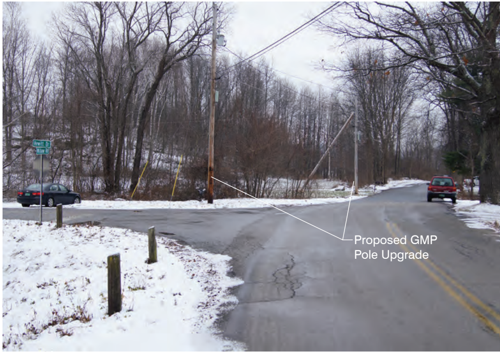
A- VIEW LOOKING WEST FROM WILLOW ROAD TOWARDS THE (3) PROPOSED GMP POLES BEING UPGRADED
