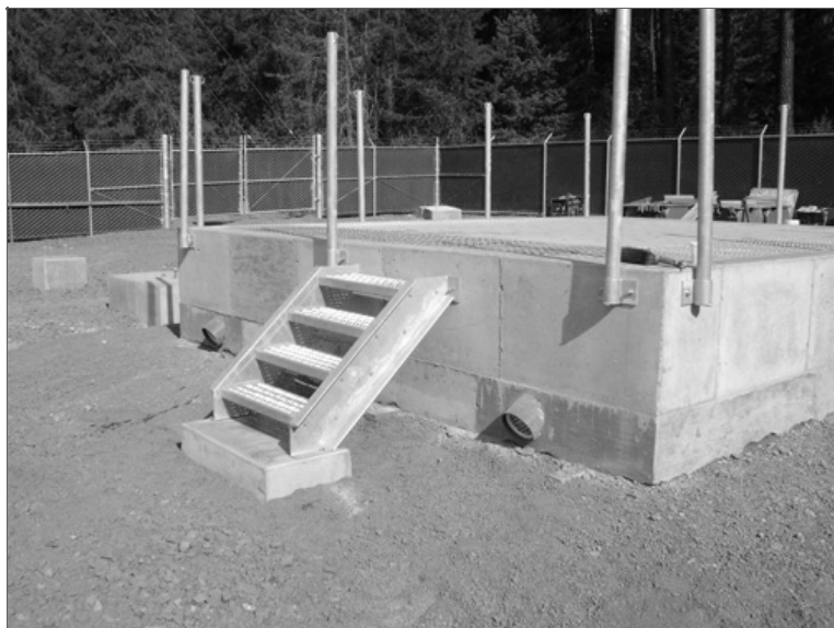
The above picture shows the Housing and Petro-Pipe installed on the correct 25 degree slope through the concrete wall.
