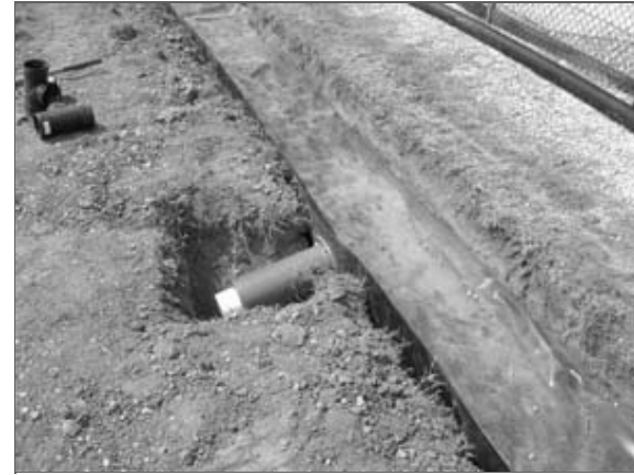
Petro-Pipe housing pipes with 4" female connectors are attached to the drainage pipe and mounted directly in the liner, forming a water-tight, oil-tight seal.
