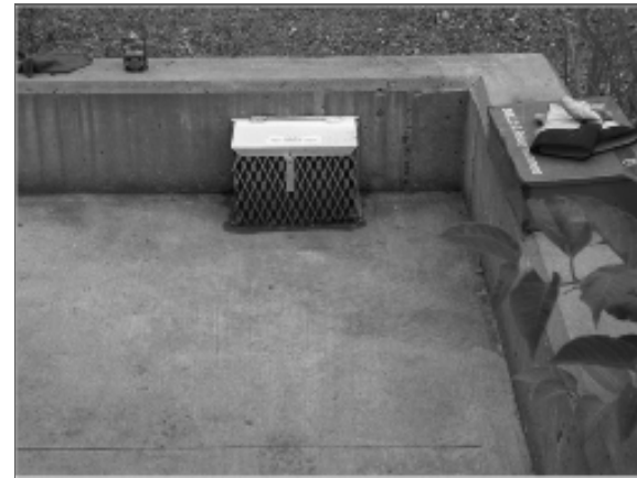
The filter basket are a great addition to the Petro-Pipe to filter out dirt and debris from entering the Petro-Pipe.
