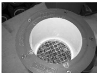
Inspect the cavity and clean out any dirt and debris. Pack firm with new floss. Replace black mesh, grate and retaining ring.
