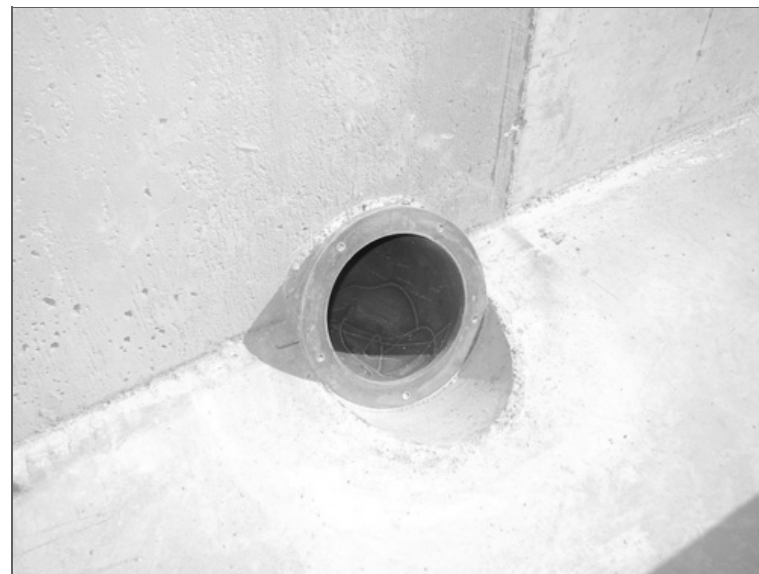
The Petro-Pipe housing is installed through the concrete at the correct angle and the concrete is cut out allowing all the water to enter the Petro-Pipe
