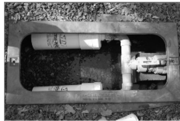
The filter basket are a great addition to the Petro-Pipe to filter out dirt and debris from entering the Petro-Pipe.
