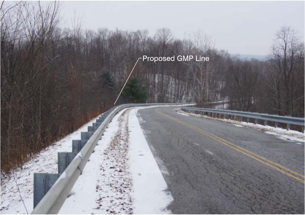
H - VIEW LOOKING WEST FROM SIDE OF HEWITT DRIVE TOWARDS THE PROPOSED GMP LINE UPGRADE
