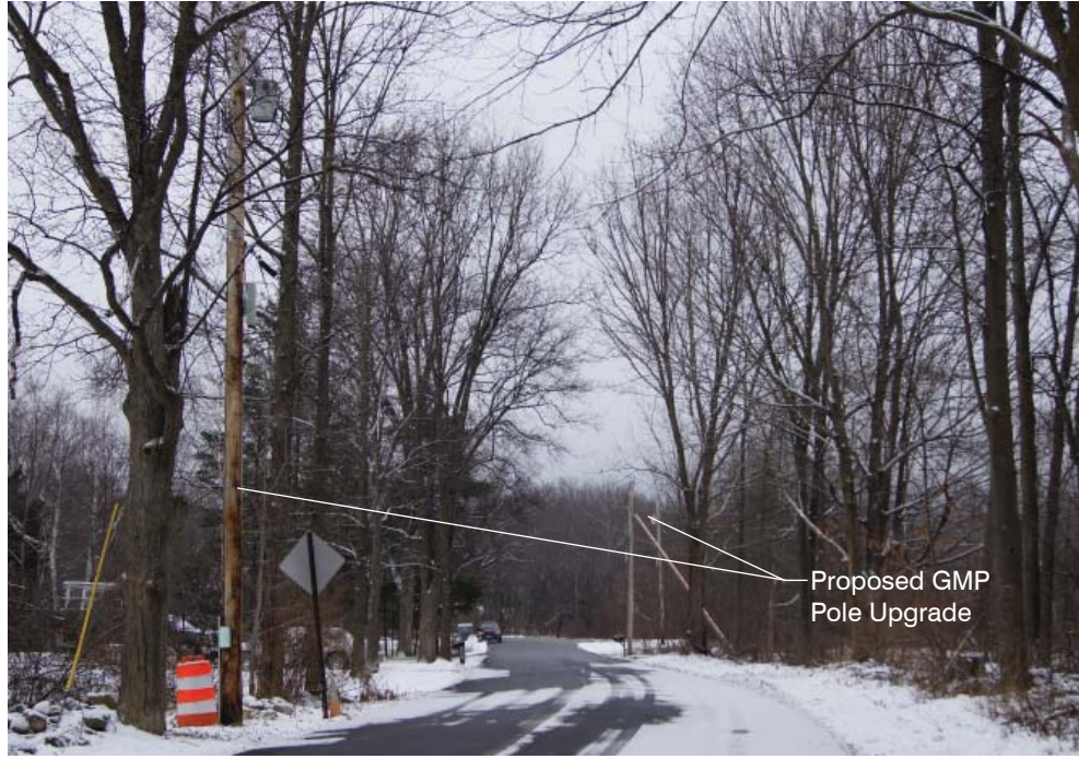
C - VIEW LOOKING EAST FROM THE END OF PAVED AREA ON WILLOW ROAD TOWARDS THE (3) PROPOSED GMP POLES BEING UPGRADED
