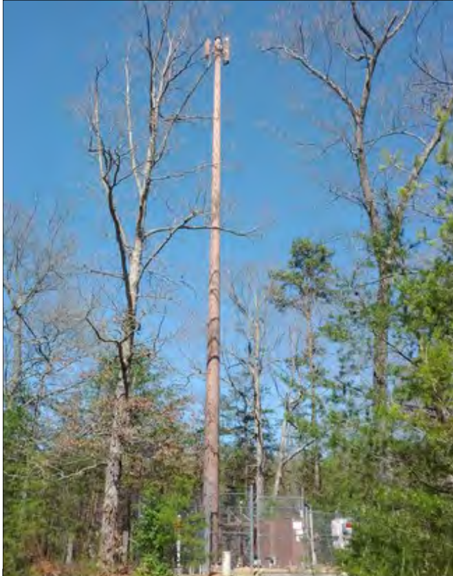
Narrow profile monopole towers such as this one tend to be less visually intrusive than larger lattice towers and towers with widely spaced arrays of antennas. “Stealth” towers designed to appear as trees or other landscape features can be effective, but only if they appear as natural parts of their surroundings.
