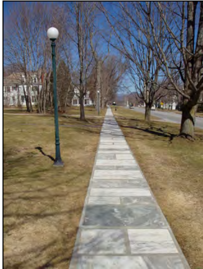
Reconstructed marble sidewalk in Manchester village.
