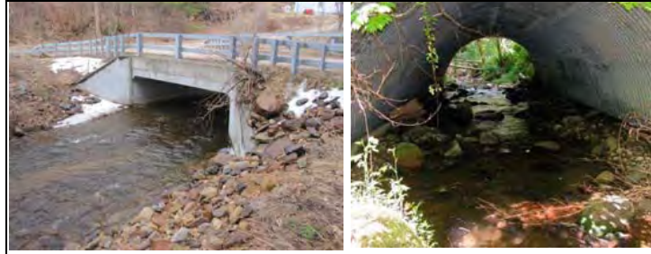
These culverts are large enough to handle flood flows; the depth and speed of water within the culverts provides suitable conditions for movement of stream-dwelling organisms.
