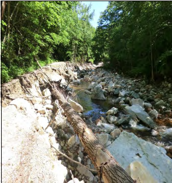
Tropical Storm Irene, in 2011, caused massive damage to the Roaring Branch in Sunderland and to the adjacent Kelley Stand Road (remnant of the road pictured above on the left side of the photograph).
