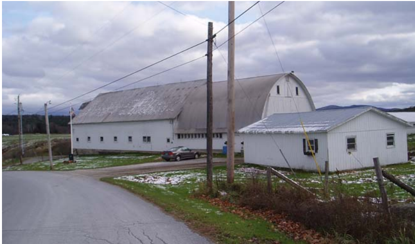
Site 14. McNall Farm barns, view looking easterly from McNall Road.
