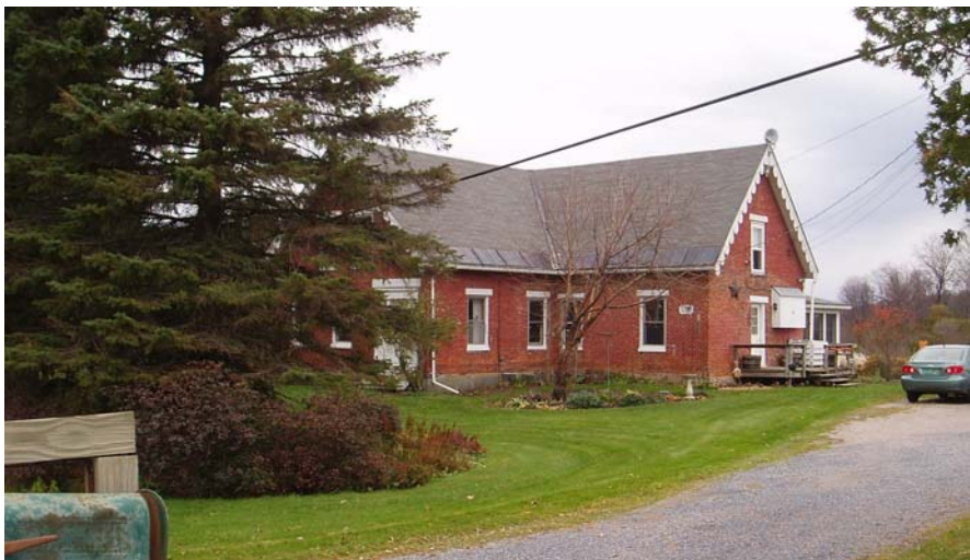
Site 16. Harvey Klein House (SR 0410-6), c. 1865, site #1, view looking northerly from Westford Road, Milton, approximately 1.6 miles from the Project.
