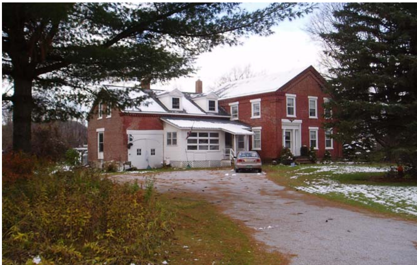
Site 21. The Brush Place (SR 0410-7), c. 1860, North Road, Milton, view looking northwest, approximately 1.1 miles from the Project.
