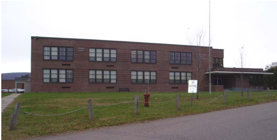
Bellows Free Academy, 1943, view looking west, just outside Fairfax Village Historic District.
