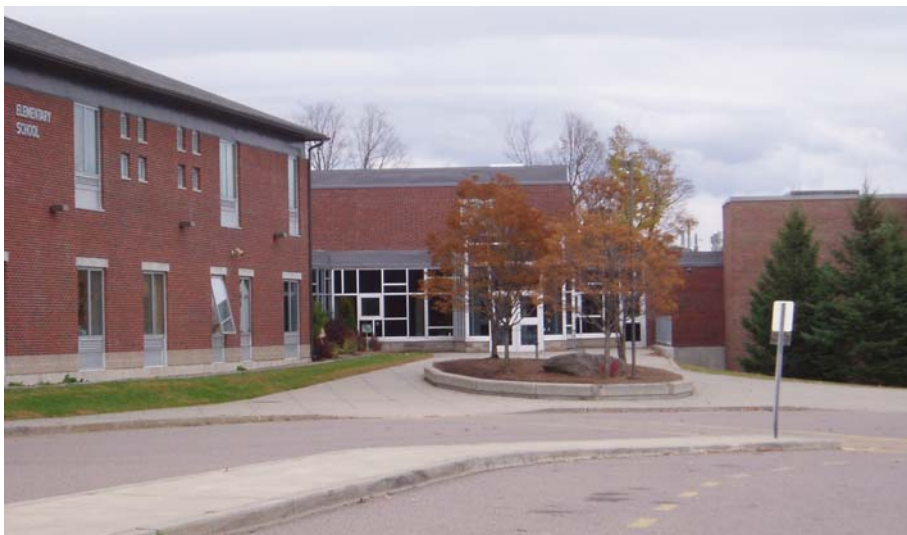
Bellows Free Academy, view looking east of modern additions behind 1943 section.
