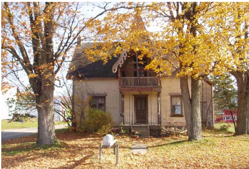
Site 20. Devino farmhouse, view to east from North Road.
