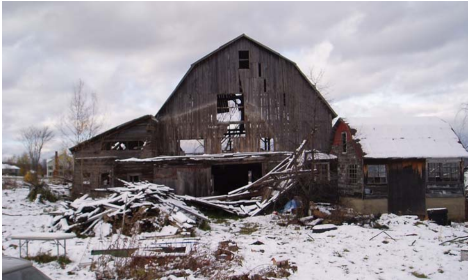
Site 15. Villado Barn, view looking northerly.
