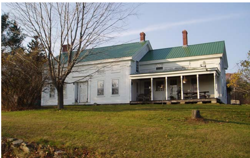
Site 23. Hathaway-Morgan House (SR 0608-17), c. 1840, Dee Road, Georgia, view looking north.
