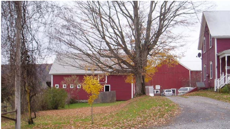
Site 9. Orton-McNall Farm barns, Route 104 north of Fairfax village, SR 0604-53, view looking westerly.
