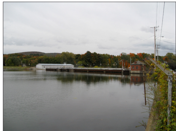
Route 7 - Arrowhead Mountain Lake with dam in background, Milton
