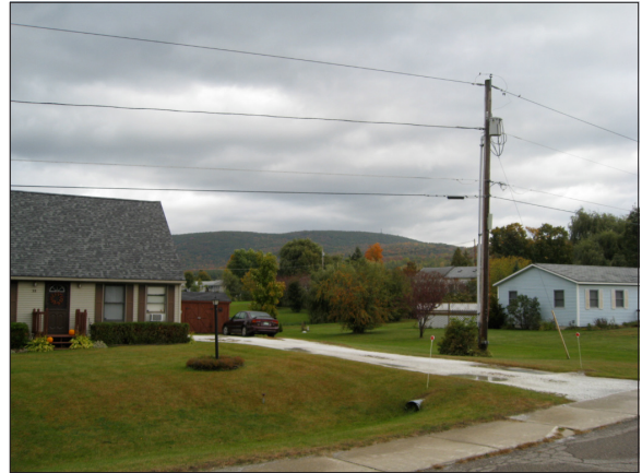
Utility lines through Quarry Lane Development, Milton
