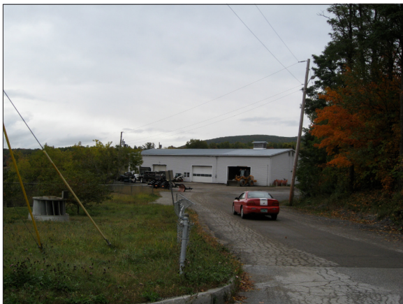
Heart of Milton Village at Ice House Road
