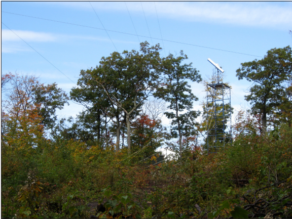
Existing equipment on Georgia Mountain, Milton
