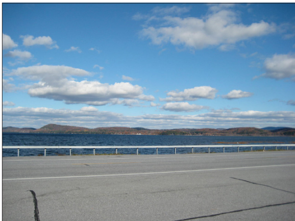
View across Sand Bar Bridge between South Hero and Milton
