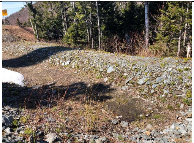
Photograph 12. Representative view of existing LS-C16.
