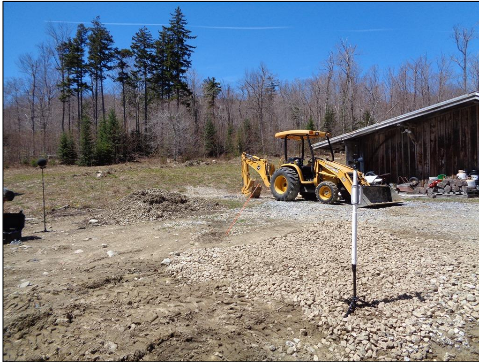
Figure 10. Site C, View to Northwest
