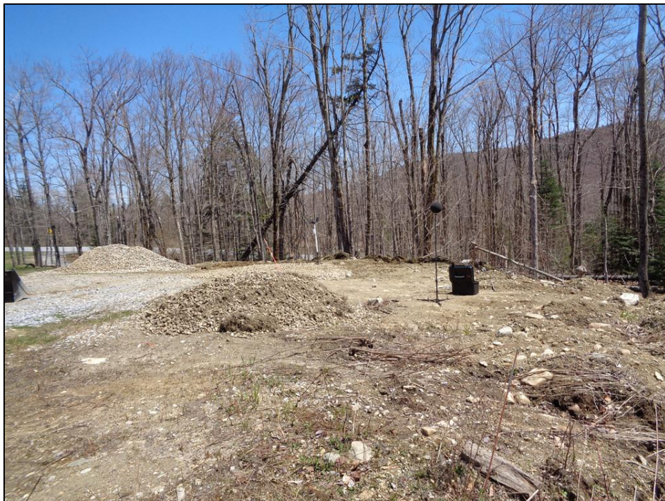
Figure 11. Site C, View to East
