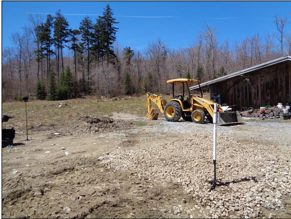
Figure 10. Site C, View to Northwest
