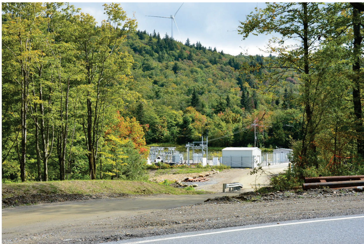
Figure 1: View taken from Route 8 looking along clearing for a new access road and storm water pond at the base of the eastern ridge. (September 7, 2017)
